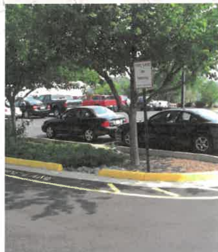
In this Virginia parking lot, traffic islands are designed with curb-cuts and a porous drainage medium to allow runoff to collect and infiltrate.
