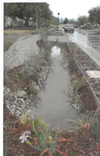
Stormwater flows through a curb inlet into a bioswale on Elmer Street. The water infiltrates into the soil within a day, preventing breeding mosquitoes.
