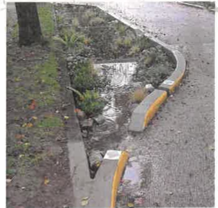
A landscaped curb extension calms traffic and captures and infiltrates street runoff in Portland, Oregon.
