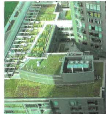
A green roof absorbs rainwater, reduces energy costs and offers wildlife habitat in urban Portland, Oregon.
